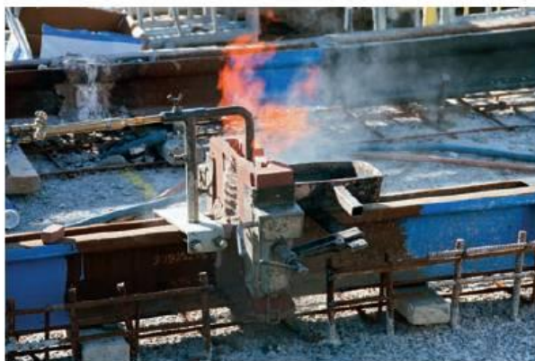
Figure 1.10 The thermit process is used to weld together the steel rails of railway tracks.
