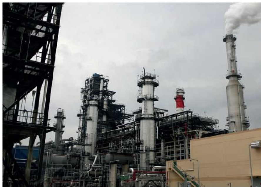
Figure 14.18 Alkenes are produced by the cracking of long-chain alkanes (see section 13.3). Crude oil is heated and passed through these catalytic cracking towers.
