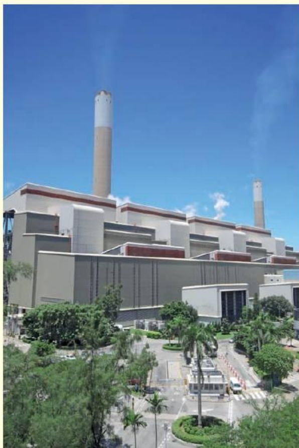
Figure 5.4 A coal-burning power station. Coal has the highest energy density of the fossil fuels, giving out 76 kJ of energy for each \text{cm}^3 of coal burnt.
