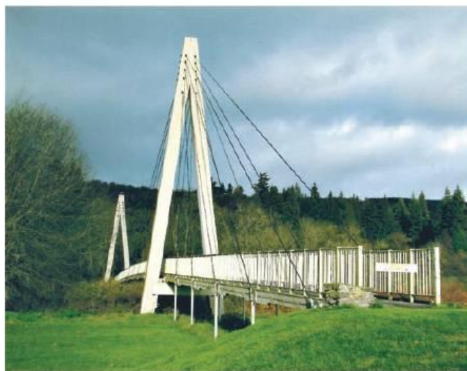
Figure 28.12 The Aberfeldy footbridge is made from glass-reinforced polyester. Its cables are made from Kevlar
